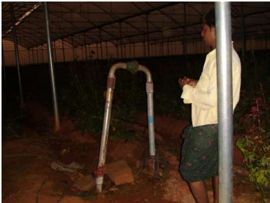
Bore Well within Greenhouse
