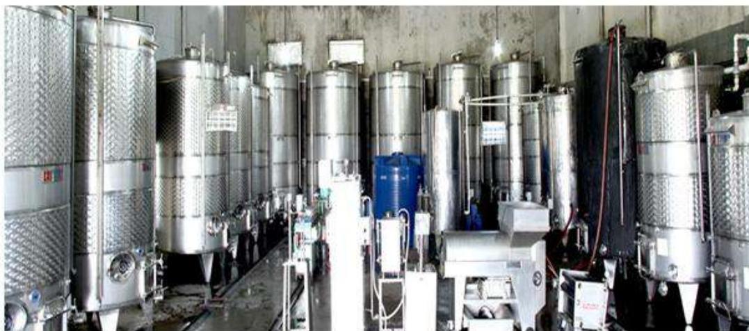
Overview of M/s Vijaya Durga Wine Industry and Storage Tank
